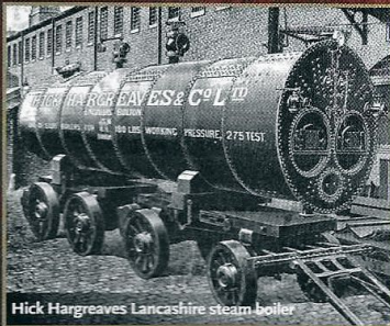
Hick Hargreaves Lancashire steam boiler
